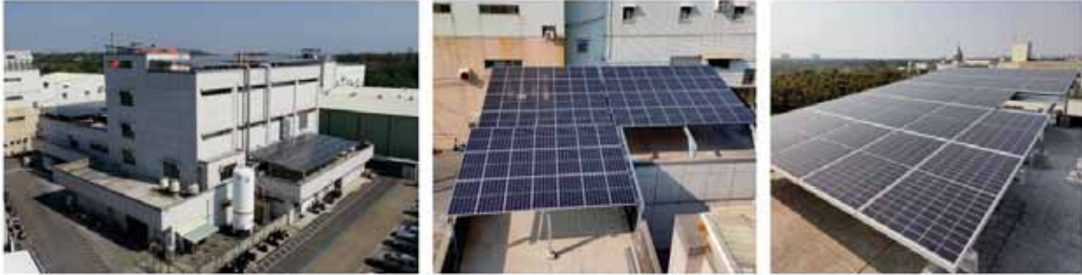
Note: Green Energy Facility Construction at MiMTW in Tainan, Taiwan.
